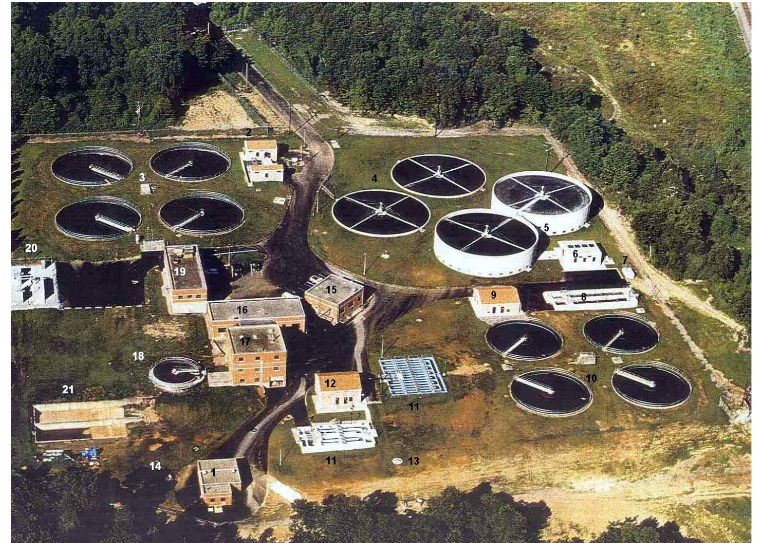
1. Main Pump Station, 2. Grit Removal Buildings, 3. Primary Clarifiers/Sludge Drawoff Pit, 4. Trickling Filters, 5. Oxidation Towers, 6. Oxidation Tower Pump Station/Meter Pit, 7. Oxidation Tower Valve Recirculation Pit, 8. Solids Contact Tank, 9. Polymer/Blower Building, 10. Secondary Clarifiers, 11. Chlorine Contact Tanks, 12. Hypochlorite Storage Building, 13. Effluent Sampling Shed, 14. Influent Sampling Shed, 15. Operations Building, 16. Press Garage, 17. Incinerator Building, 18. Sludge Thickener, 19. Maintenance Garage, 20. Electrical Station, 21. Ash Lagoon
