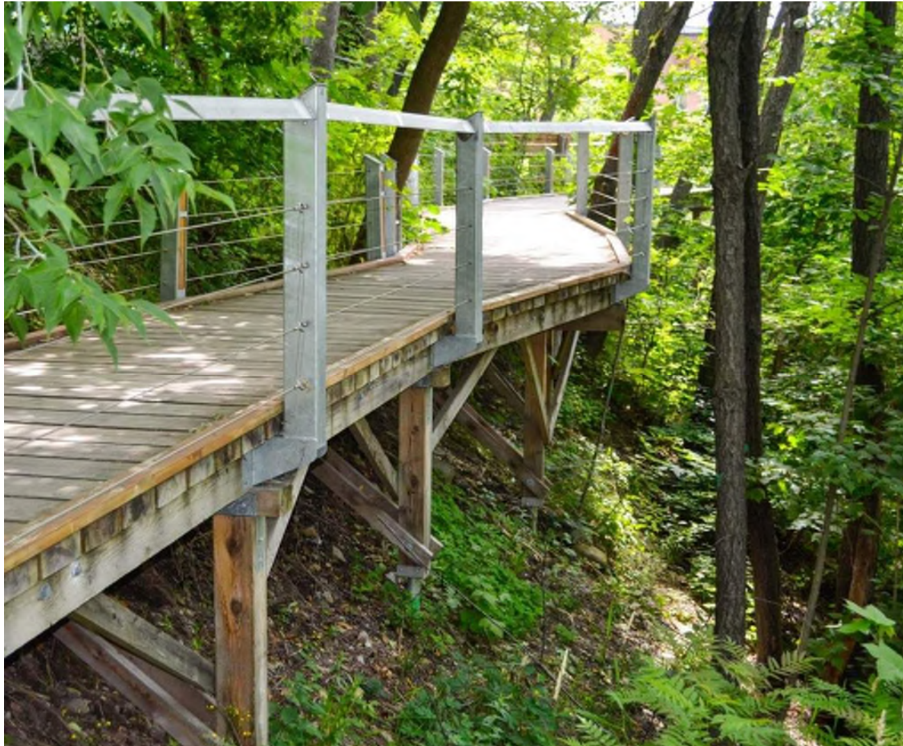
Timber Boardwalk on Helical Pile Foundations Image courtesy of TechnoMetalPost
