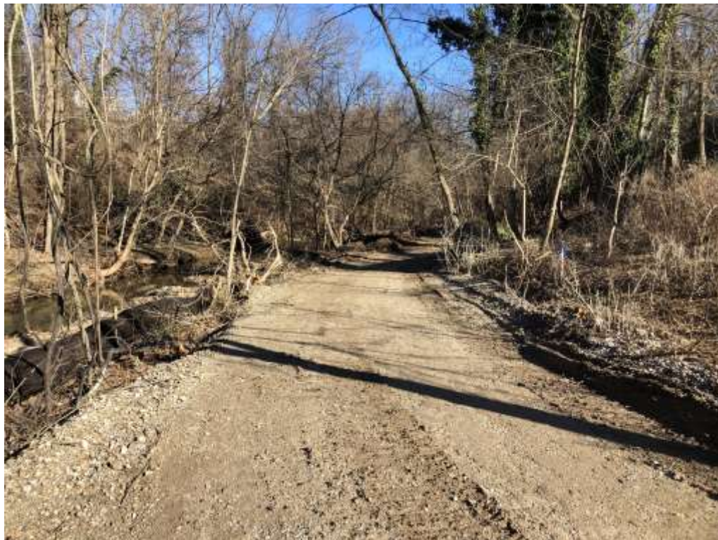
Segment 2B – East view of trail with clearing and stone base placed
