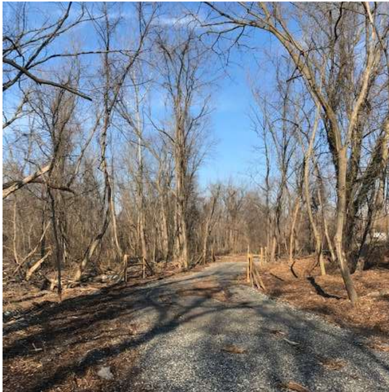
Segment 3A – Trail with clearing and base stone complete
