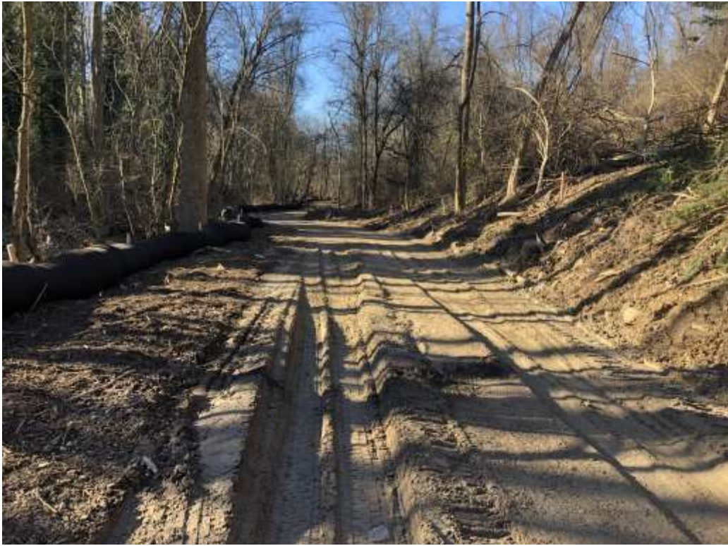
Segment 2B – Looking west with trail clearing & stone base placed
