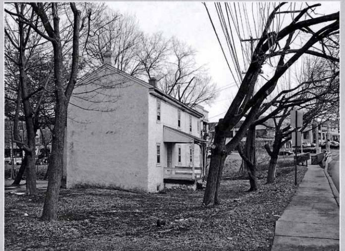
Elwood Powell House Farmhouse surrounded by commercial development Allendale Road off 202, Upper Merion Township
