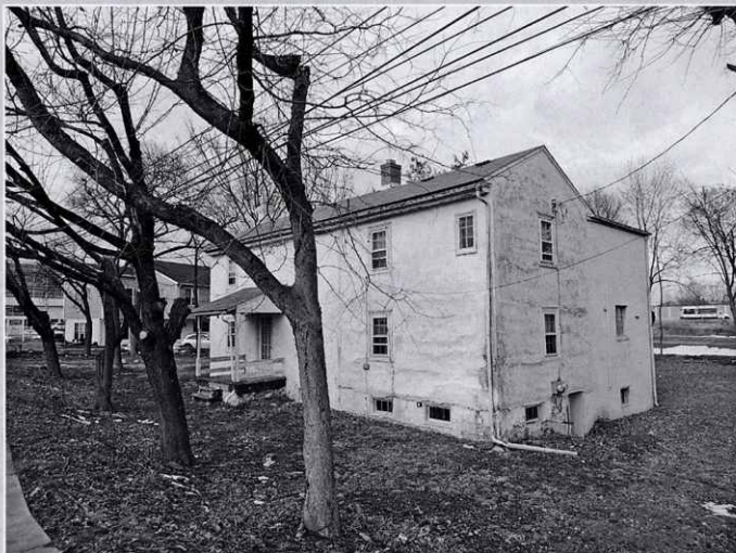
Elwood Powell House Farmhouse surrounded by commercial development Allendale Road off 202, Upper Merion Township
